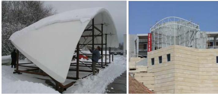
Figure 37. Fitting of the roof segments (lower wing of 'The Library') at Holland Composites in March 2005. Figure 38. Building site in Tel Aviv zoomed in on 'The Library' with the truss and columns already installed.
